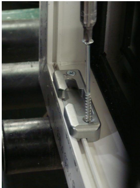
Figure 29: Replacing tilt & turn keeper screw to anchor sill
