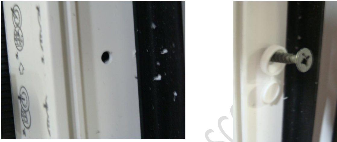
Figure 27: Installation hole (left), and with screw and cover (right)
